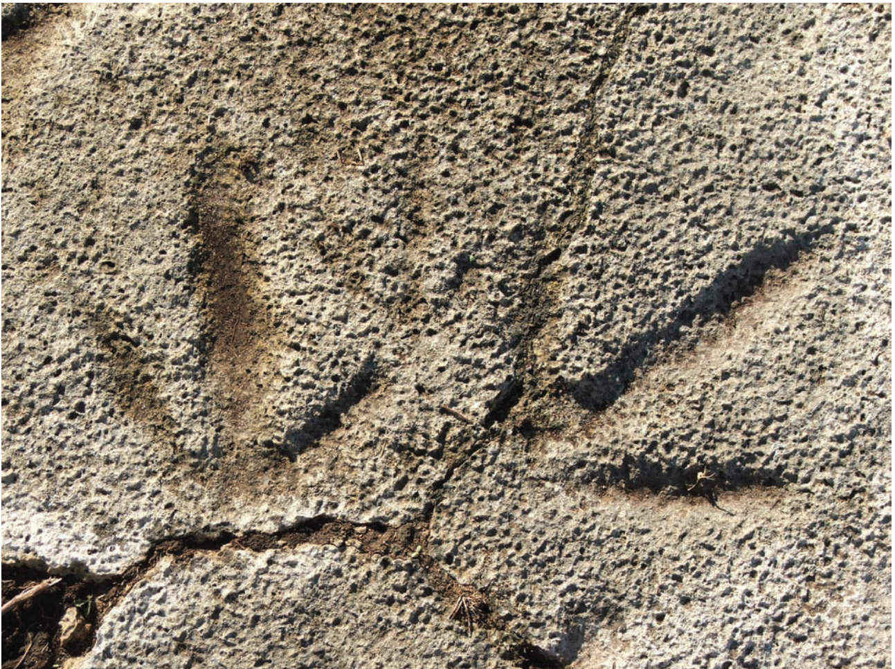
Figure 7. Vermicular surface of the rock showing vegetation attracting cracks (Panel E02)
